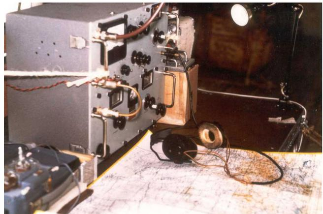
*The BW7A receiver lashed in position on the plotting table inside the aircraft (with pieces of string!)*
